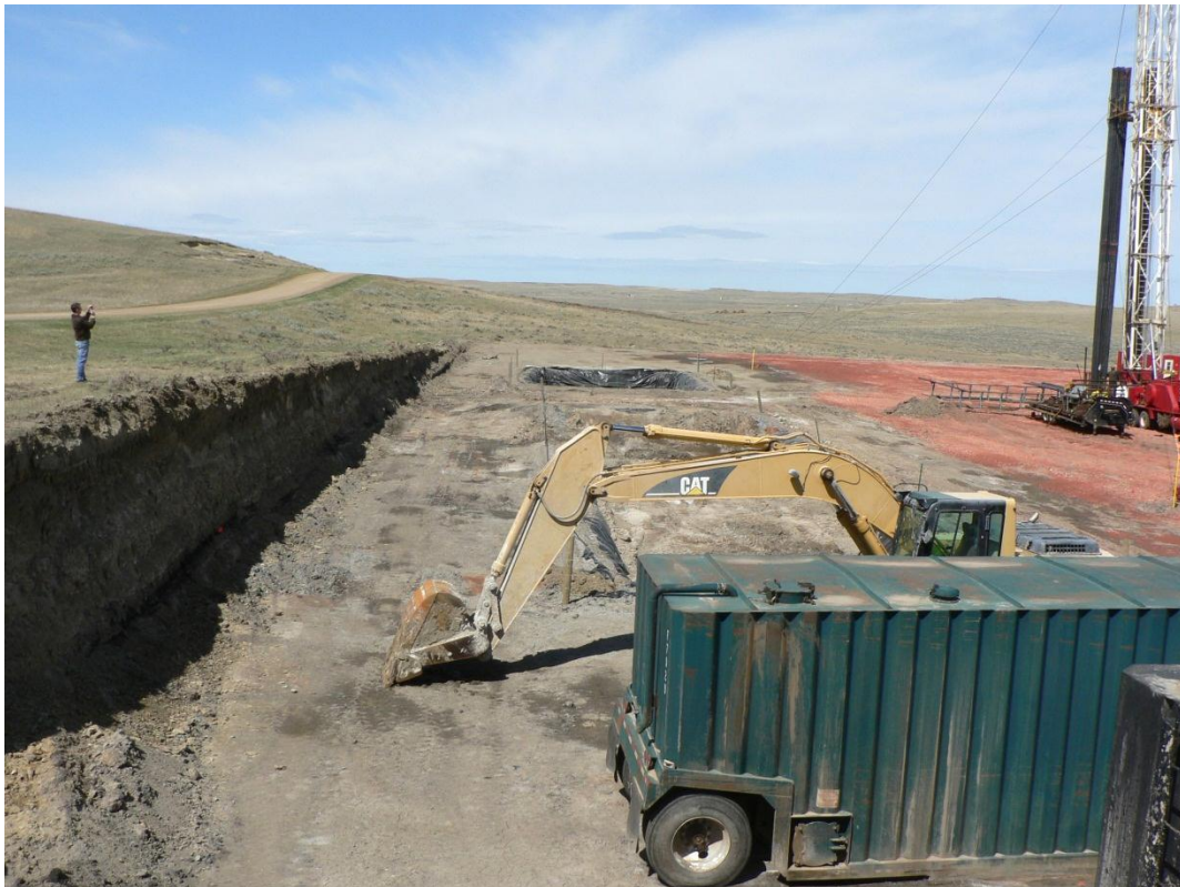
The site of a recently drilled well on the Niemi ranch, including the excavation completed for the pad. The work-over rig present on site was installing production tubing.
