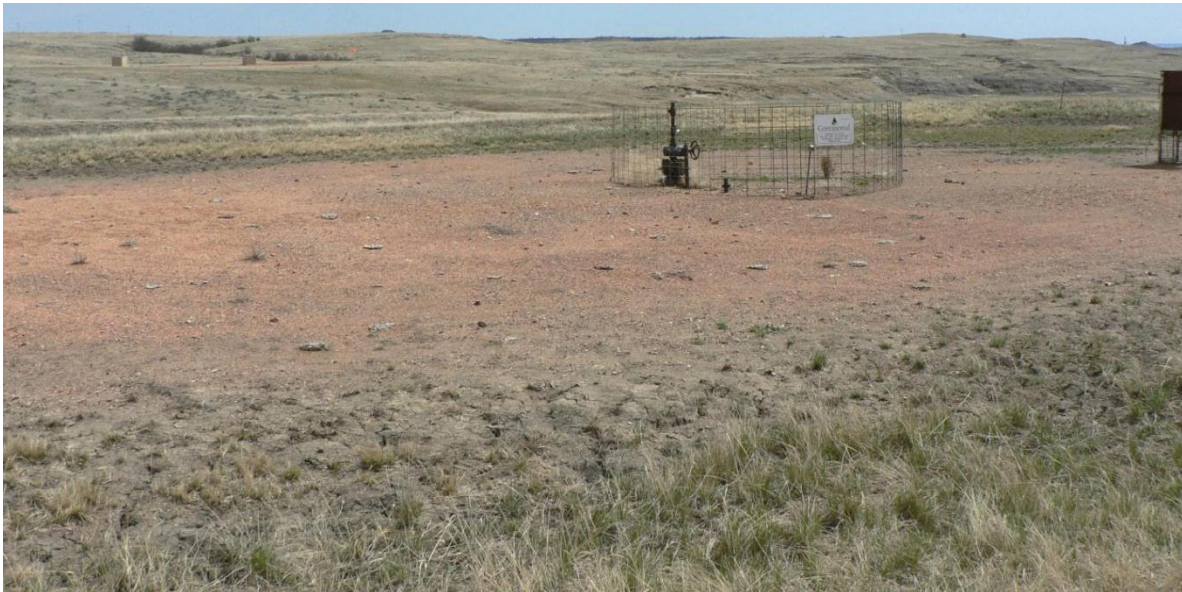
A well on the Jim Clarkson ranch in Harding County. This vertical well was drilled in 1991 and produced oil until 2004. It is currently in Temporarily Abandoned (TA) status pending final plugging and abandonment.
