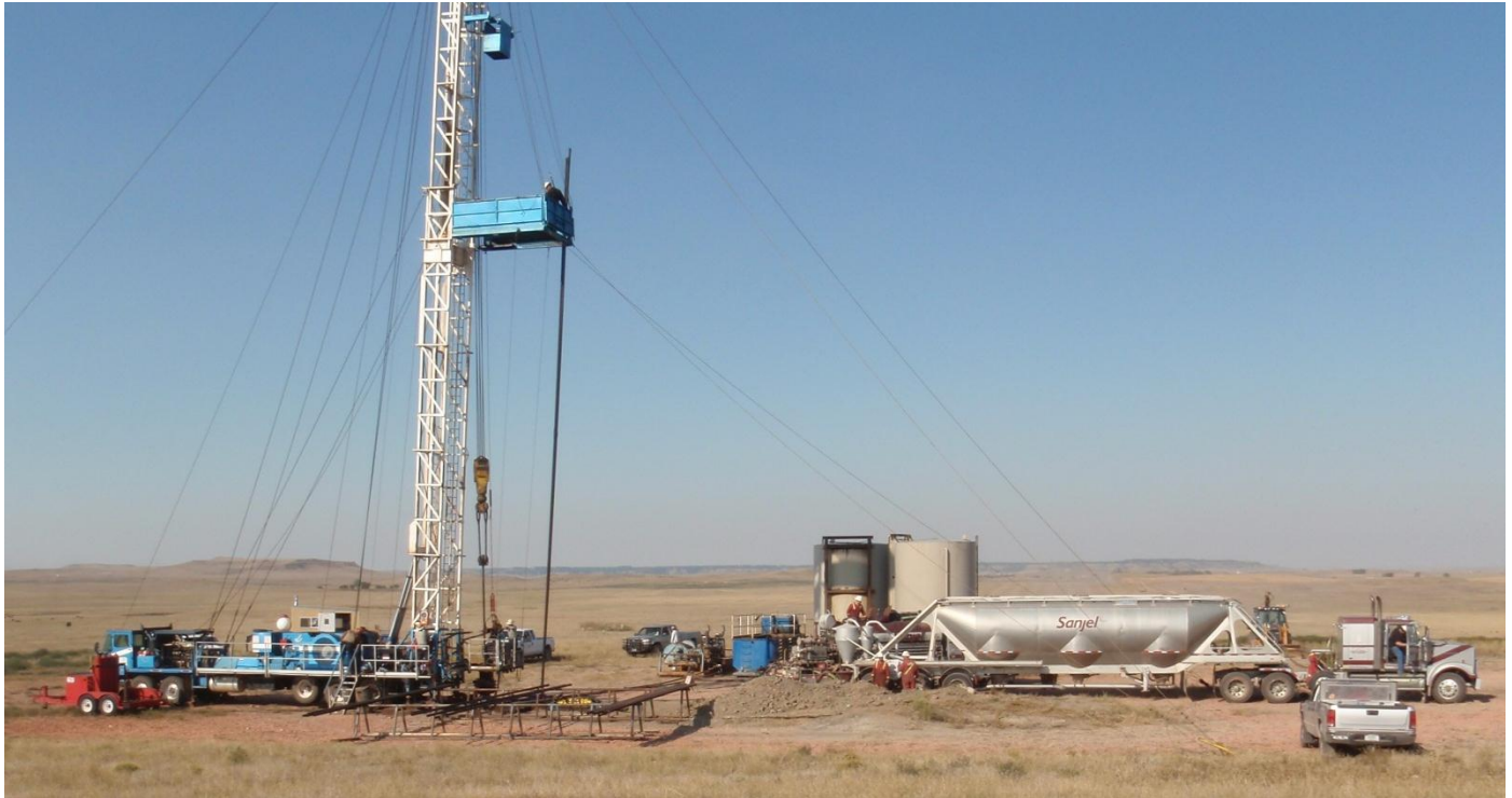
Plugging Crew at Continental Resources, Inc.'s Beer Mug Ranch Well, Harding County
