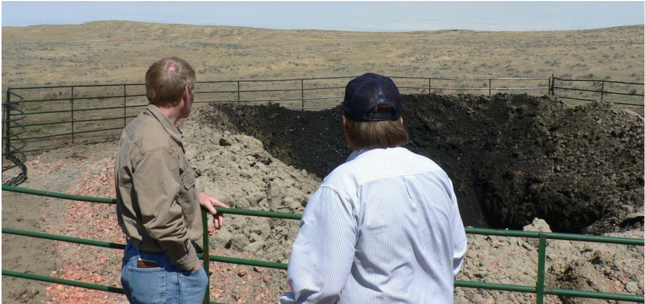
A flare pit associated with a well in the West Buffalo Red River Unit on the Niemi ranch. This well was drilled in November 2011. The black residue is from gas produced by the well, which was venting from the pipe in the flare pit. Note the discoloration of the grass downwind from the flare pipe.
